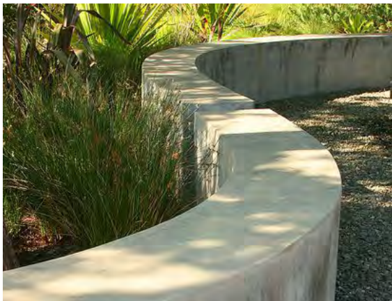
Insitu concrete wall
