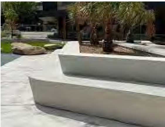
Insitu concrete terraced seating
