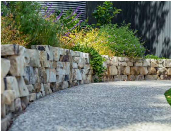
Stone retaining wall
