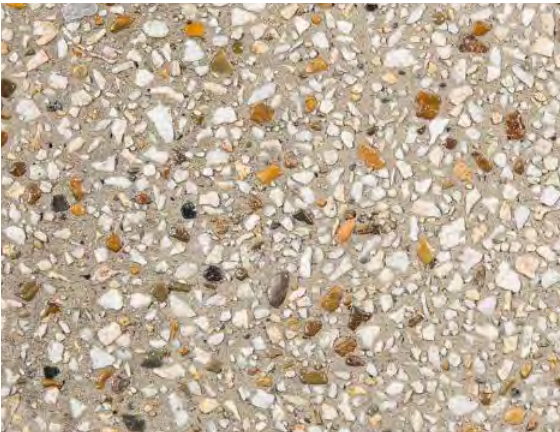
Exposed aggregate concrete
