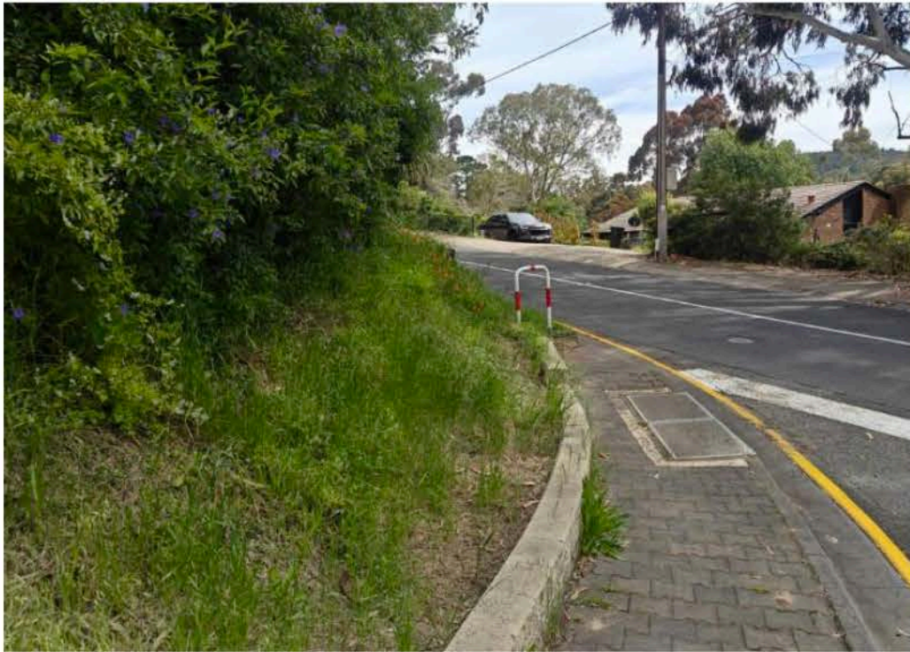
Embankment Blocking visibility at the intersection
