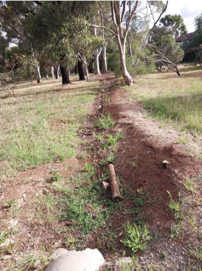
Earth berms used to direct stormwater
