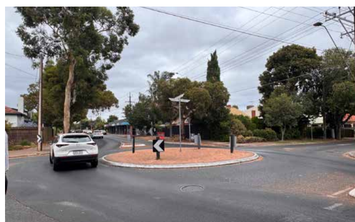
Albert Street roundabout for pedestrian safety upgrade
