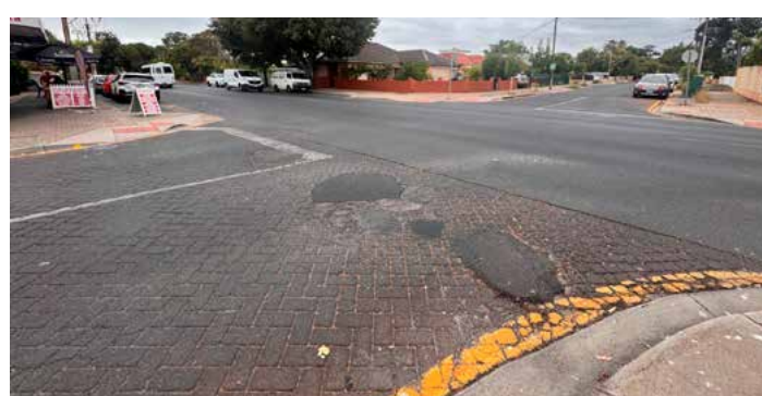
Caulfield Avenue intersection will be upgraded for traffic and pedestrian safety
