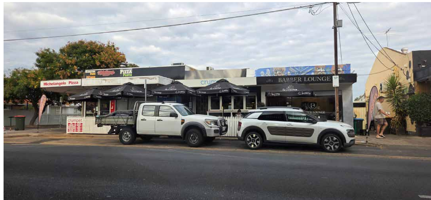
Crumpet / Caulfield Avenue Shops
