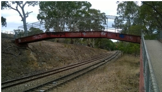
Figure 3.13: Beaconsfield Road Pedestrian Bridge over the Railway Line
